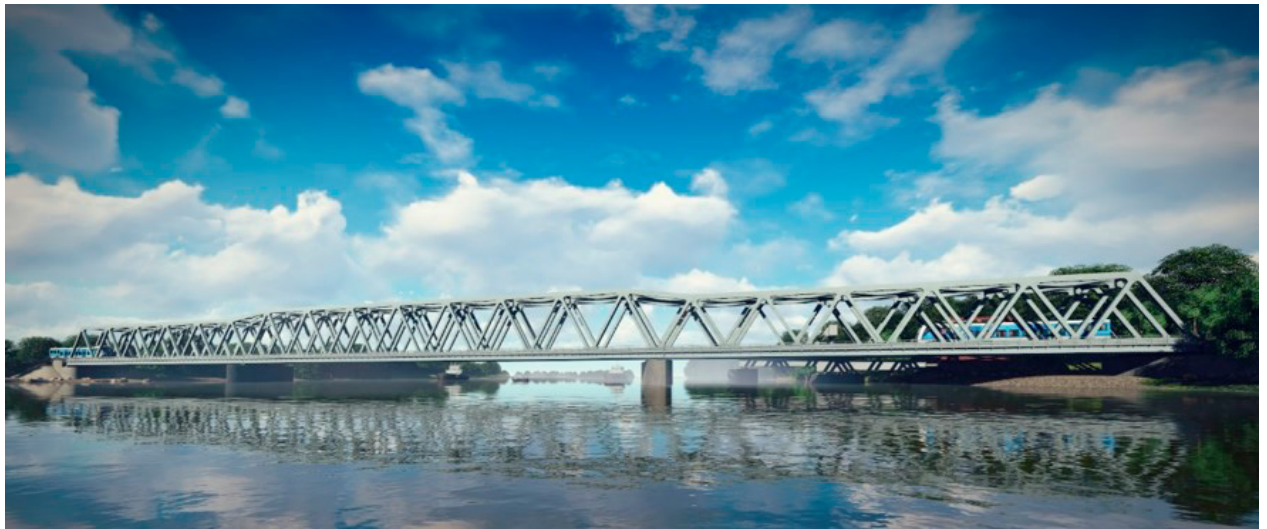
Visualisation of the new bridge
