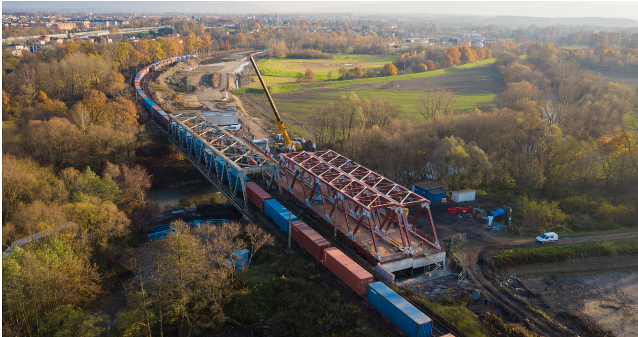
Bridge over Vistula River
