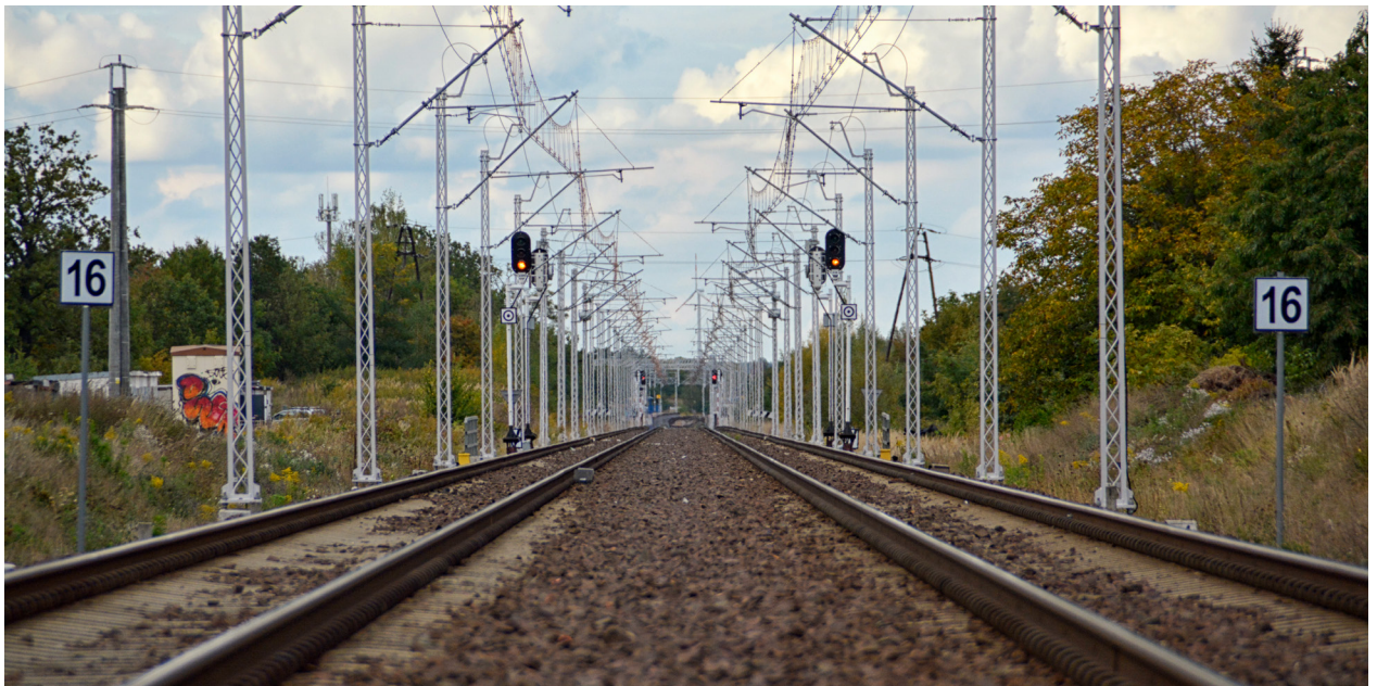
Completed electrification of the line
