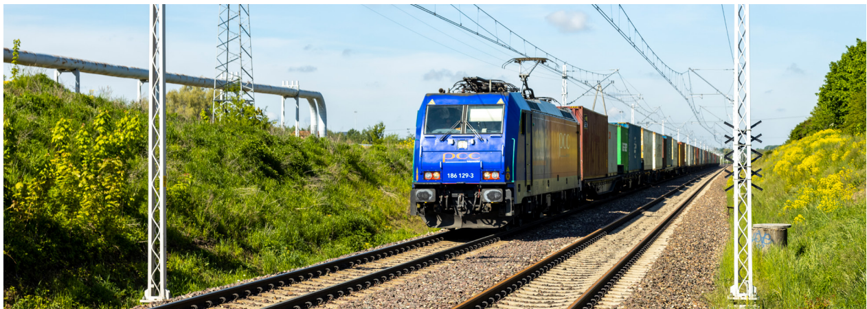
Modernised infrastructure near Kutno
