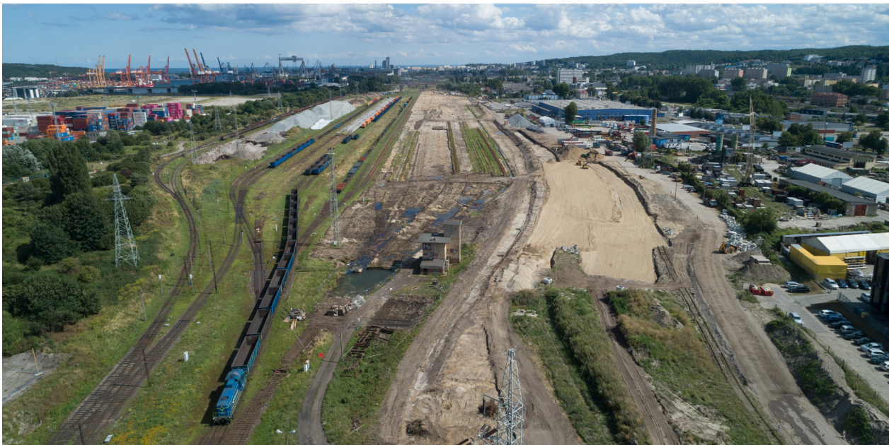
Gdynia Port station, project underway
