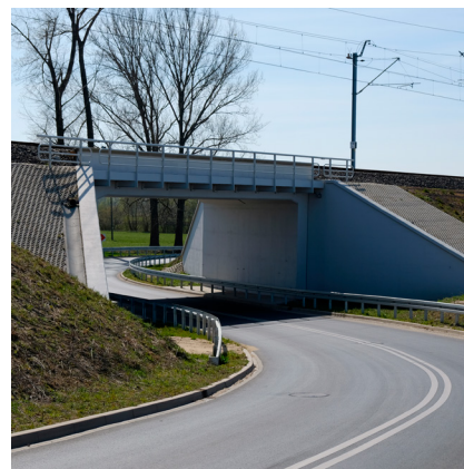
Viaduct built in Widziszewo
