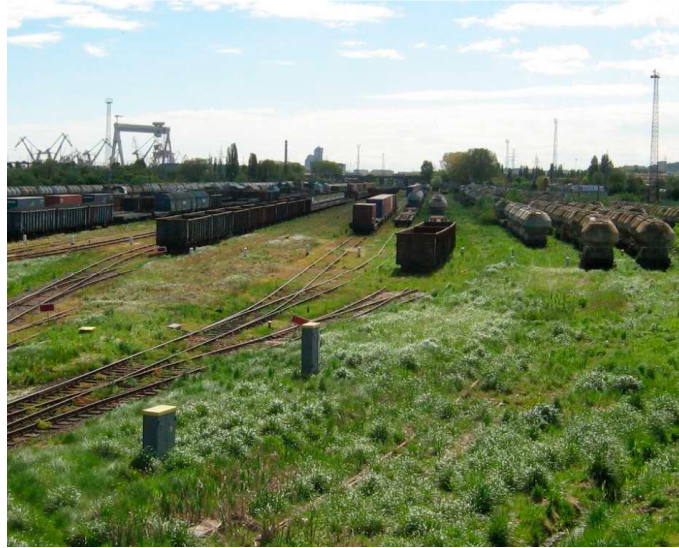
Gdynia Port station, view before implementation
