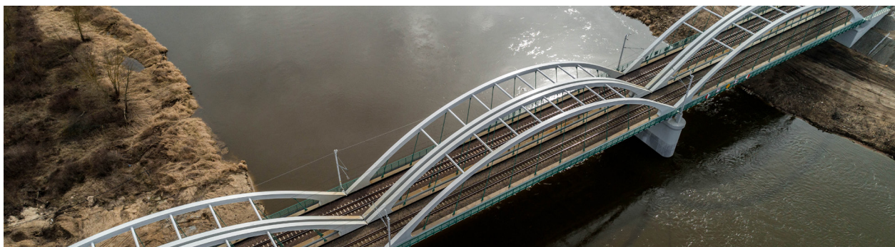
New bridge over Bug River
