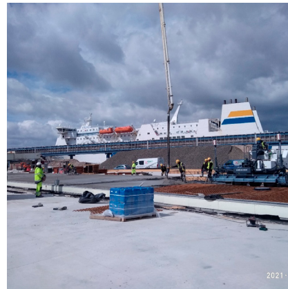
Works on the D yard
