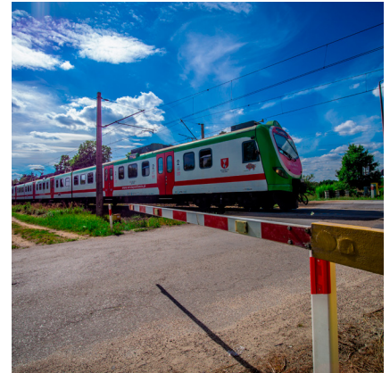
Level crossing in Trypucie, view before implementation
