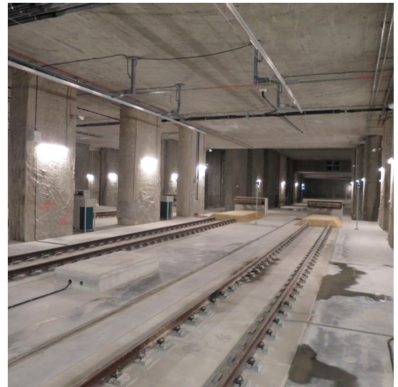
Conventional line tunnel in Łódź
