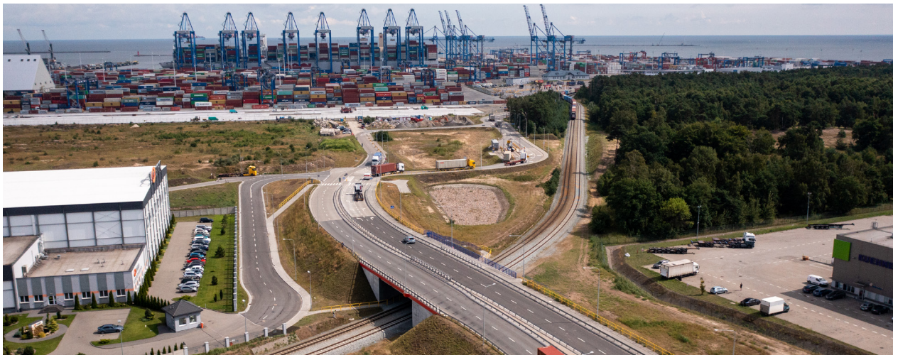
Access to DCT terminal
