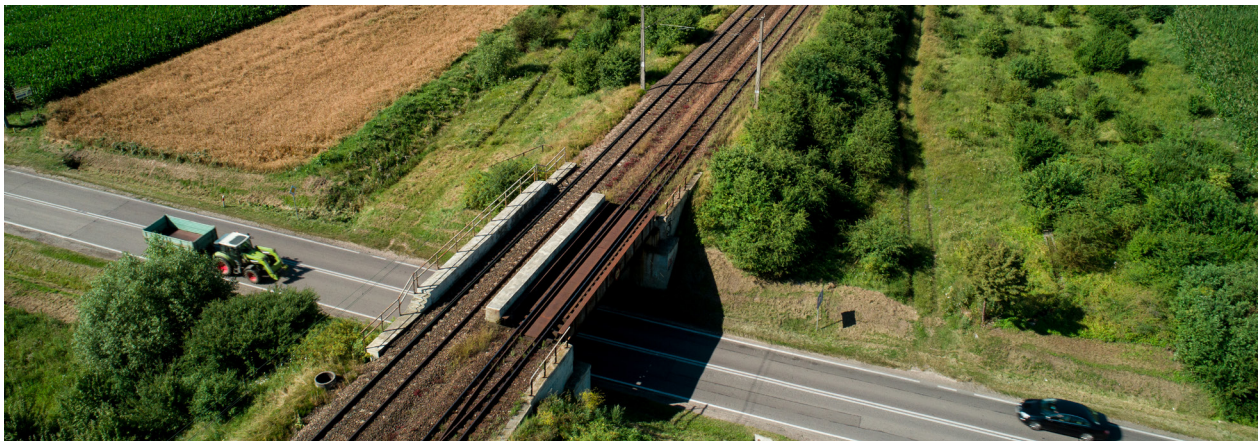
Viaduct near Czyżew, view before implementation
