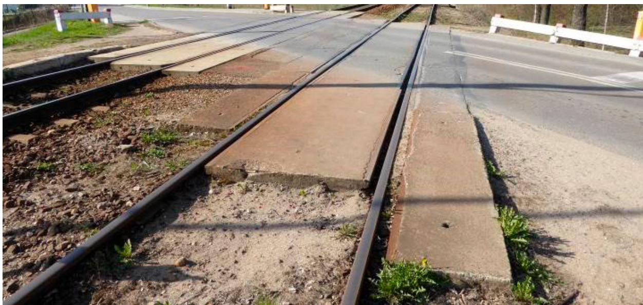
Level crossing in Ełk, view before project implementation
