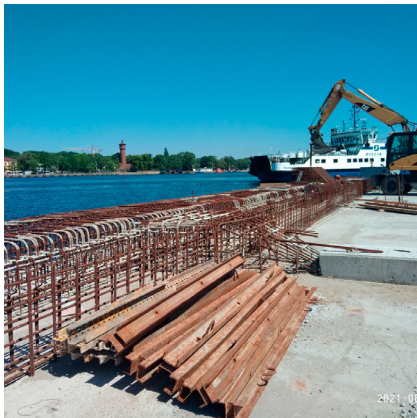
Reinforcement works on the quay
