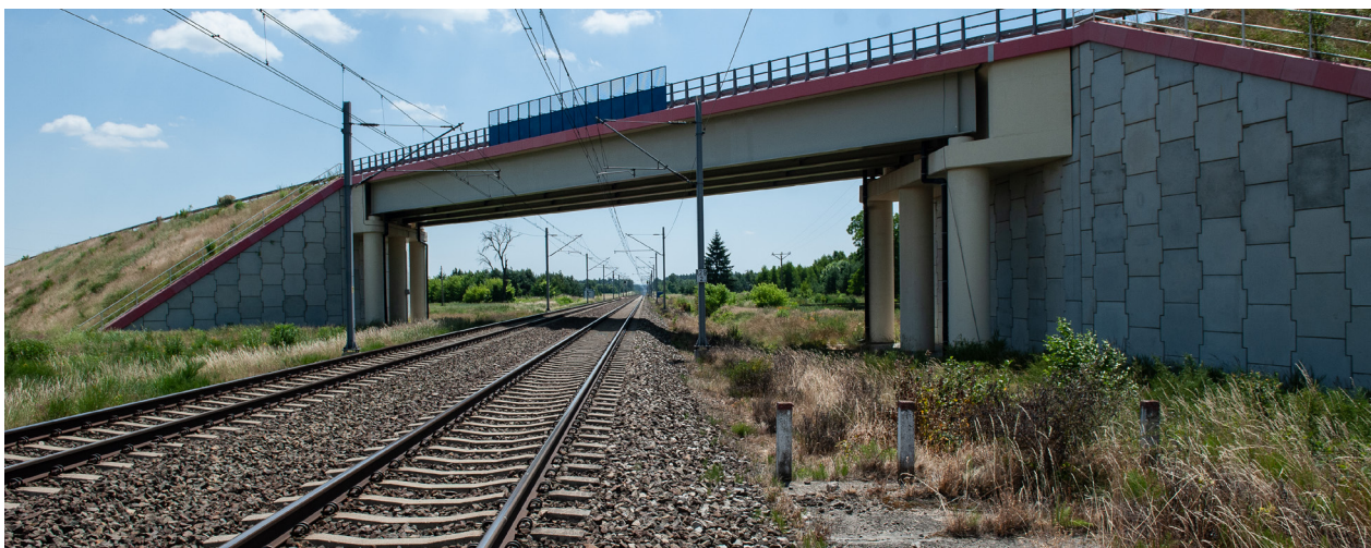
New road viaduct over CMK
