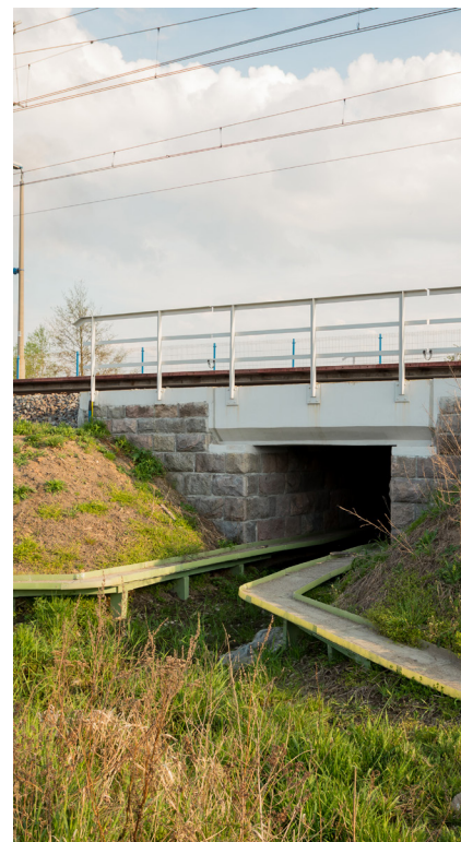
Renewed culvert in Borszewice
